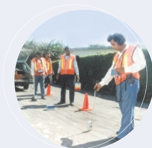
Leak Detection Works ◀
