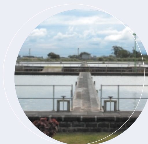
La Marie Treatment Plant ◀
